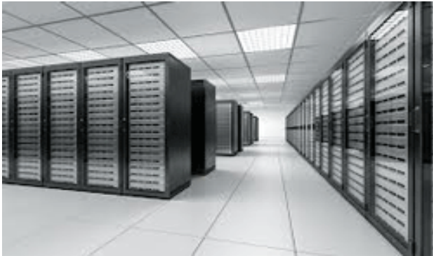
Fig.7 Stationary battery energy storage system
